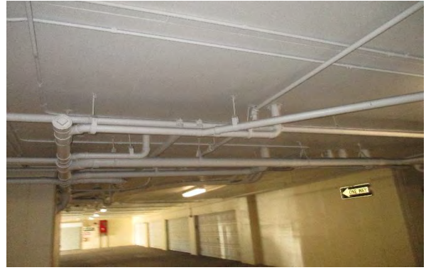
26 Plumbing Chase Overview
