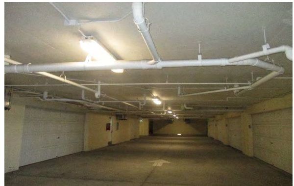
24 Plumbing Chase Overview
