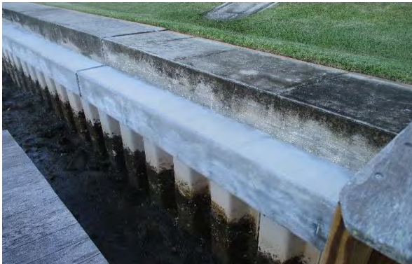
7 Retaining Wall Overview
