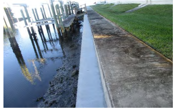
6 Retaining Wall Overview
