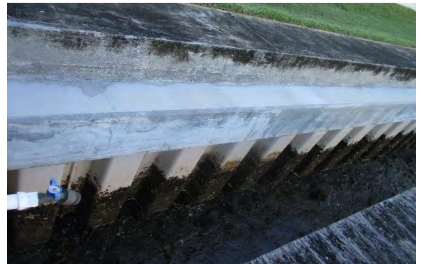
8 Retaining Wall Overview
