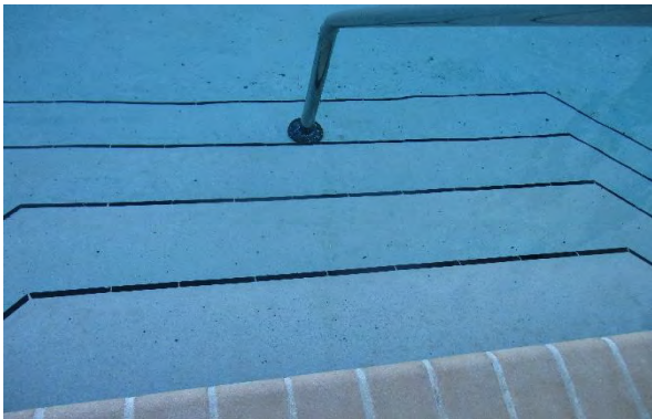
21 Pool Surface Overview
