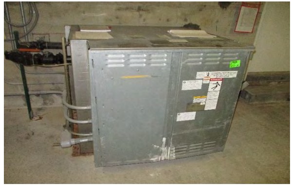
42 Elevator Motor Overview
